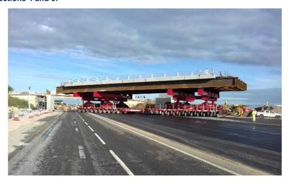
The installation of the decks of the two new bridges at Bar Hill using self-propelled mobile transporters (SPMT) was successfully completed eighteen hours ahead of schedule, by noon on Sunday 16 September. Work continues to complete the bridges and the new junction will be opened next year.
